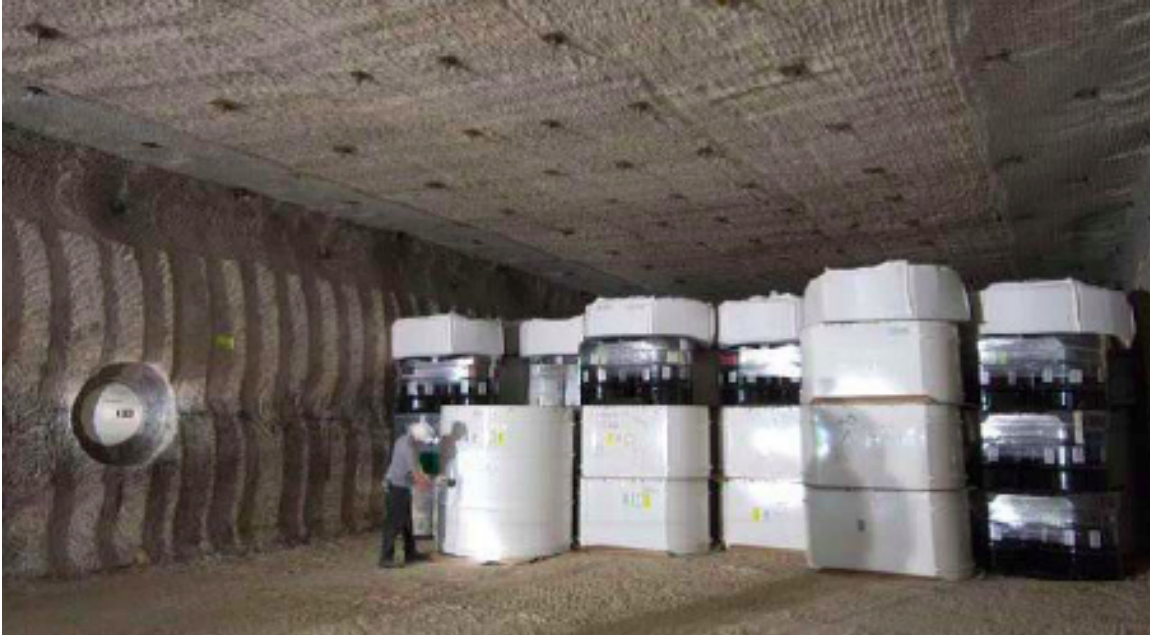
Fig. 2. Boxes of magnesium oxide desiccant are placed on top of stacks of waste containers to limit solubility of radionuclides [from Nelson, p. 9].
